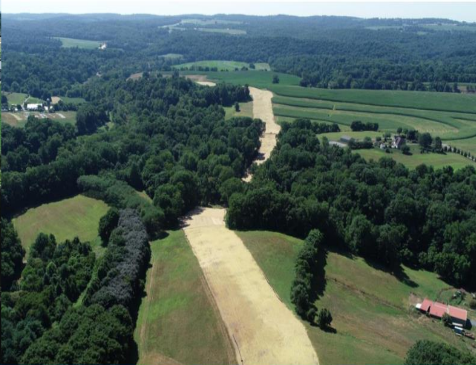
ATLANTIC SUNRISE POST CONSTRUCTION Transco Pipeline, Pennsylvania
