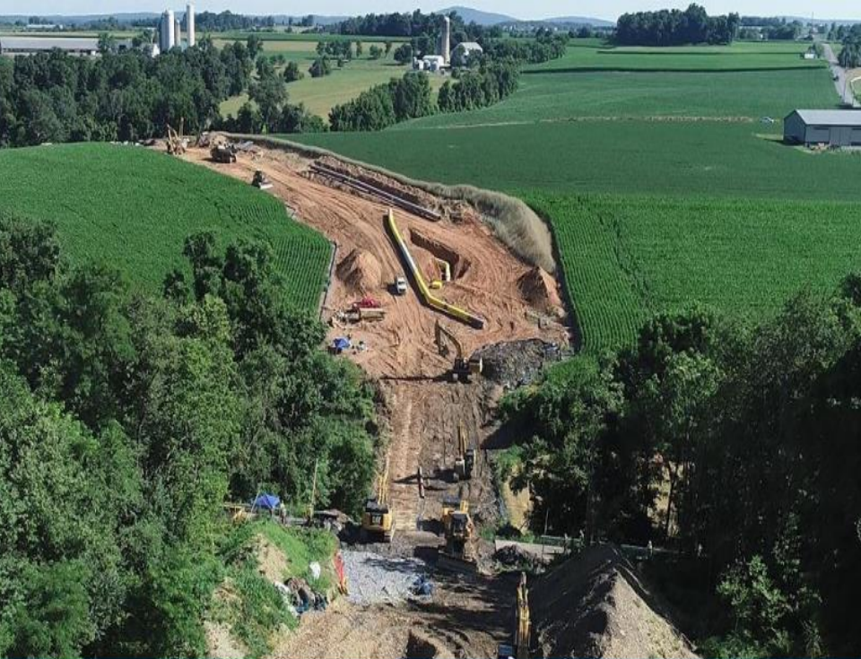
ATLANTIC SUNRISE CONSTRUCTION Transco Pipeline, Pennsylvania
