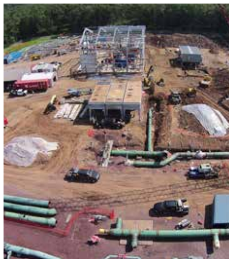
Construction at Transco Station 517 in Benton, Pa.
