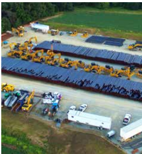
Maryland pipe yard used for Rock Springs construction
