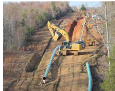
Virginia pipeline construction
