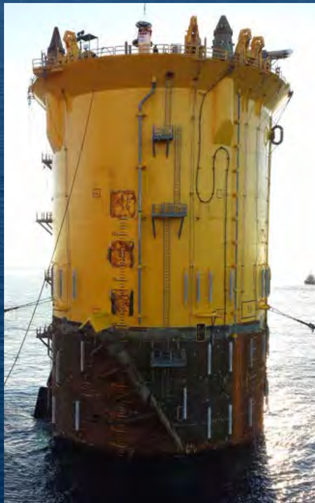
Top: Gulfstar One's topsides were set on the hull, combining the two main pieces of the Gulfstar One production system. Bottom: The Gulfstar One hull was floated into the Gulf earlier this year.
