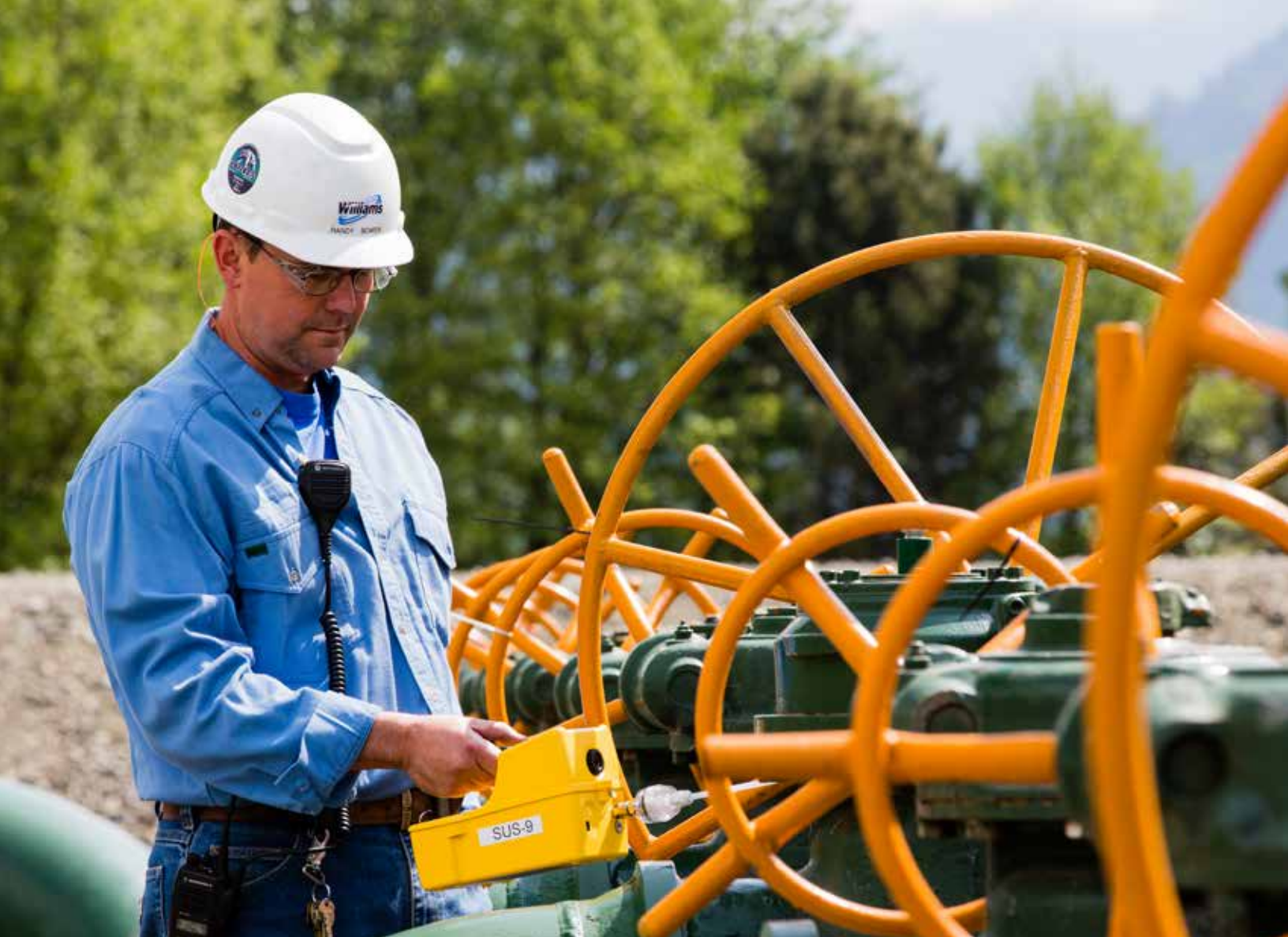
Randy Bowen, senior operations tech, performs a safety check at the Northwest Pipeline Sumas compressor station in Washington.
