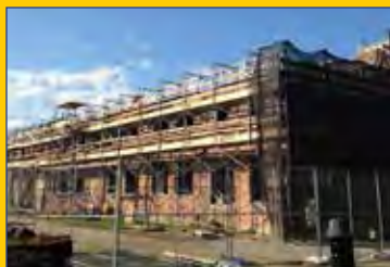
Restoration and construction efforts are ongoing in the hangar building at the Floyd Bennett Field.
