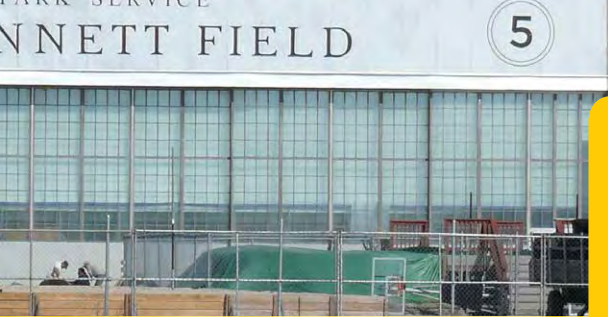
Williams is constructing a 60,000 square foot meter and regulator station inside of one of the abandoned airplane hangar buildings on historic Floyd Bennett Field in New York as part of our Rockaway pipeline project.
