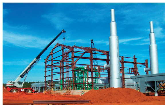
Transco Station 85 construction nears completion
